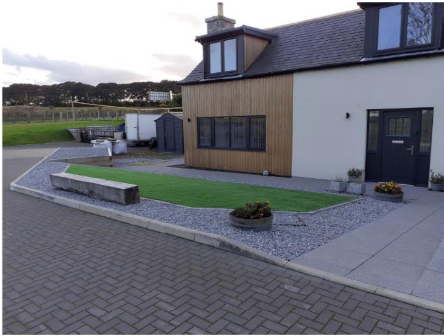
Existing Site Photograph
